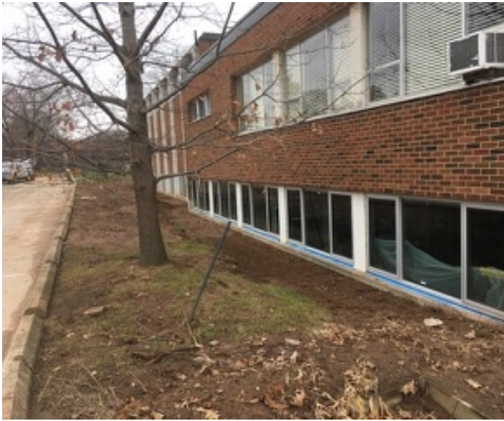
On a warm day in mid-November all windows were replaced
