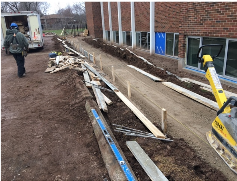
Preparation for the sidewalk to playground area
