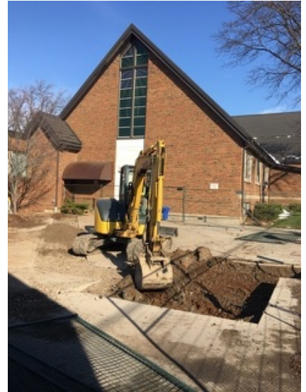
Preparation for the Transformer Vault for electrical connections.
