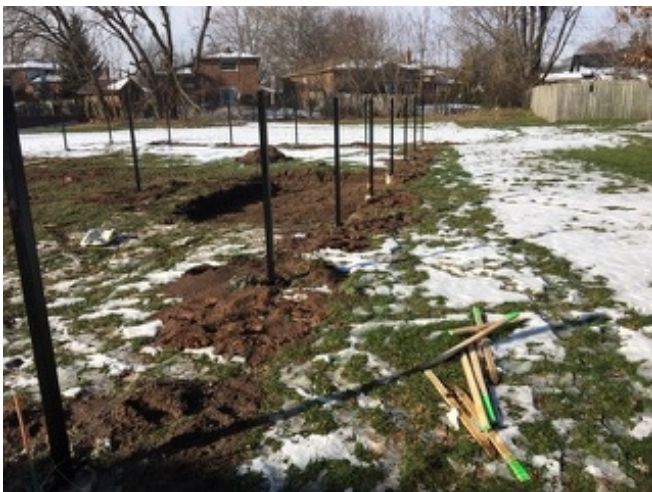
Playground fence posts in place
